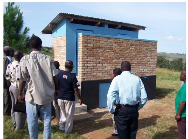
Photo 2: OSIENALA team inspecting an Ecosan Toilet constructed in a school
