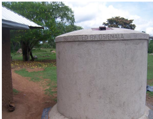
Photo 1: A ferro-cement tank constructed in a home in Kajulu
